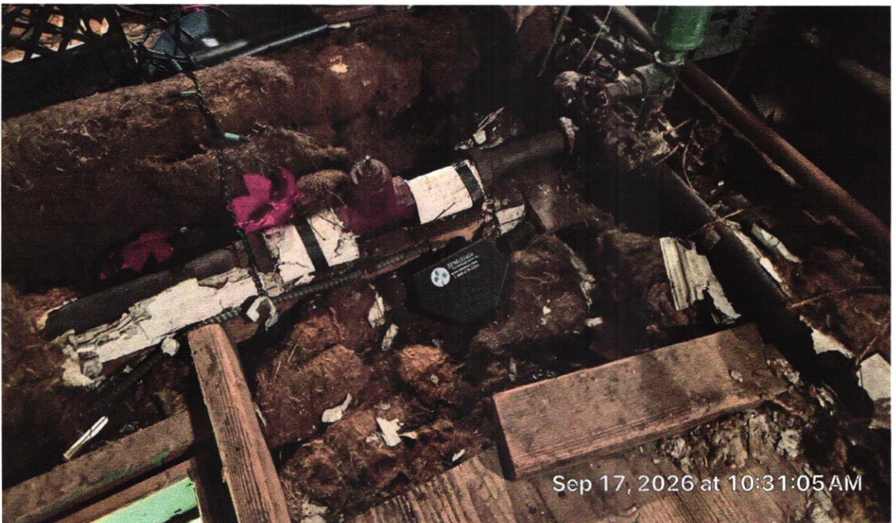
Damaged minor piping insulation around the access hatch.
