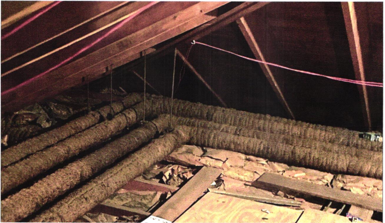
Damaged minor piping insulation around the access hatch.
